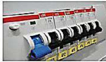
MCB - Miniature Circuit Breaker
